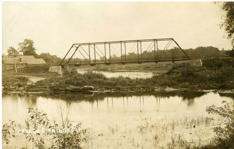
Knaggs Bridge—1856 structure with earthen impoundment
