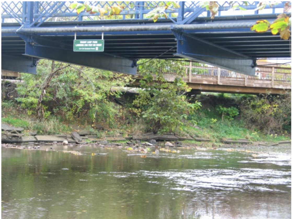
Oakwood Avenue 1876 Iron Bridge, Voight Loop Trail in Owosso
