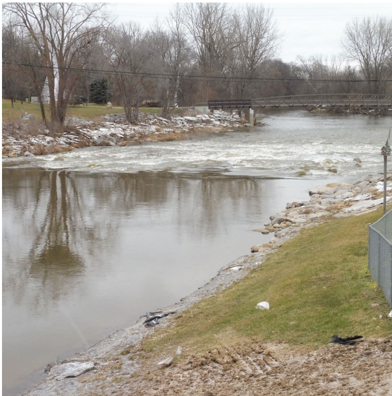
Chesaning's downtown rock ramp with landing on the right-downstream from this in-river ramp at Cole Park.
