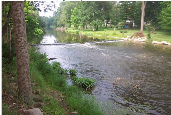
Weir at Owosso Memorial Hospital
