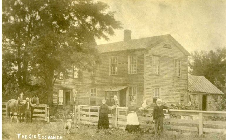
The Old Exchange – Knaggs Bridge area near Bancroft
